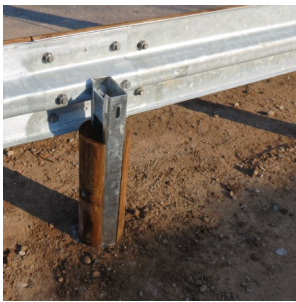
C125 steel posts with post spacing 1.33m or 2.66m
