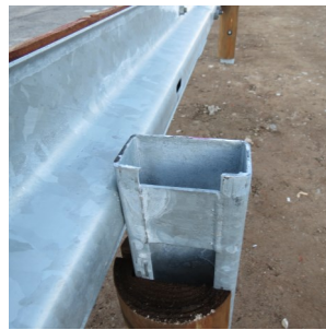
B profile Steel rail (296x4300x2.5mm) clad with four half round logs of 16cm meter
